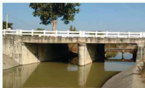
Upper Indravati Extension-Trial run
