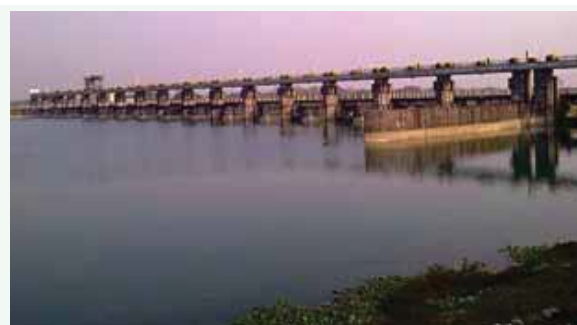
Champamati Irrigation Project (Major). at Nagdolbari Village, Dist. Chirang, BTC (Assam)
